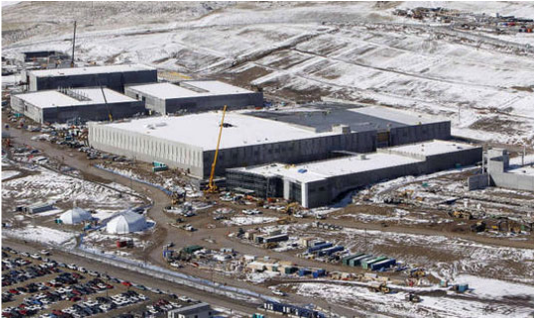
• Aerial front view of the Utah Data Center under construction - March 2012
