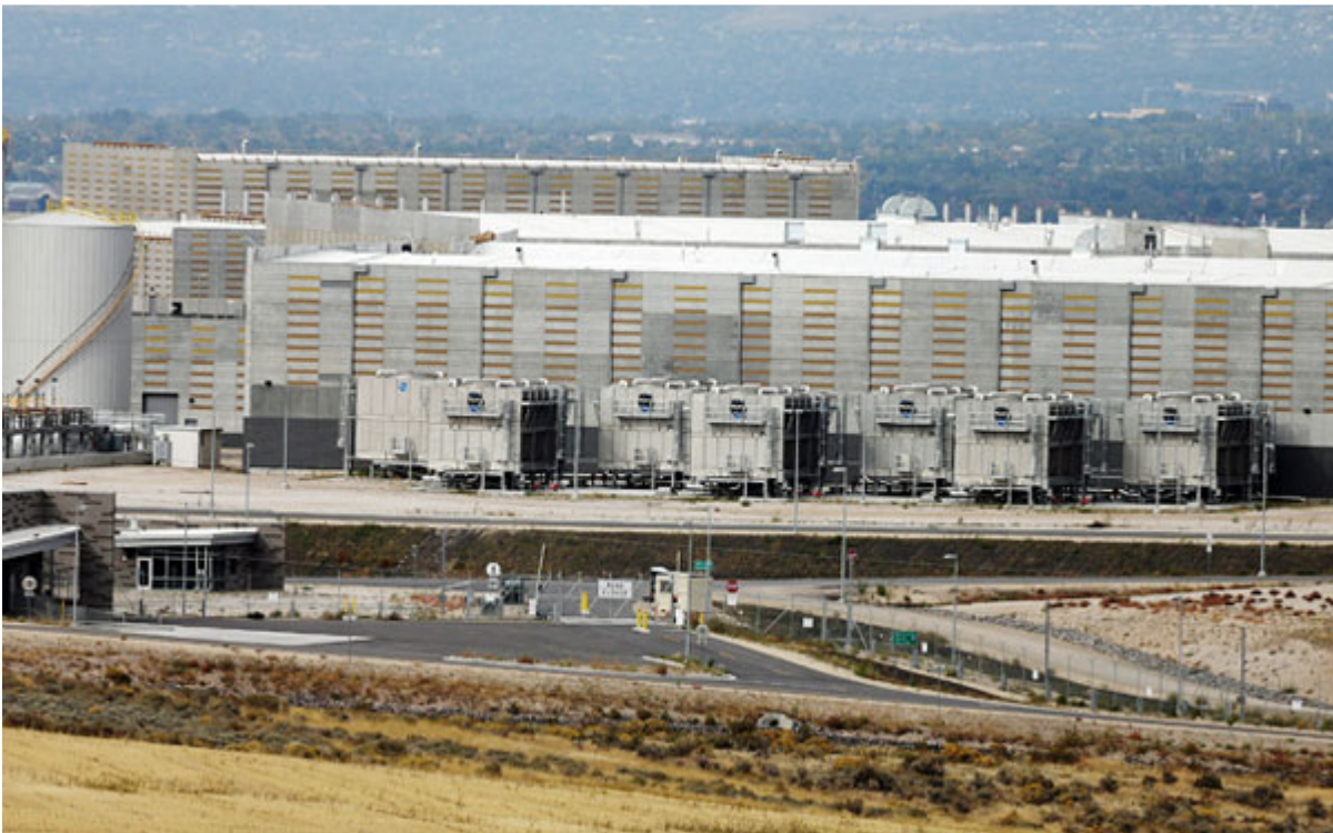
October 2013 - Southern end of the Utah Data Center facility
