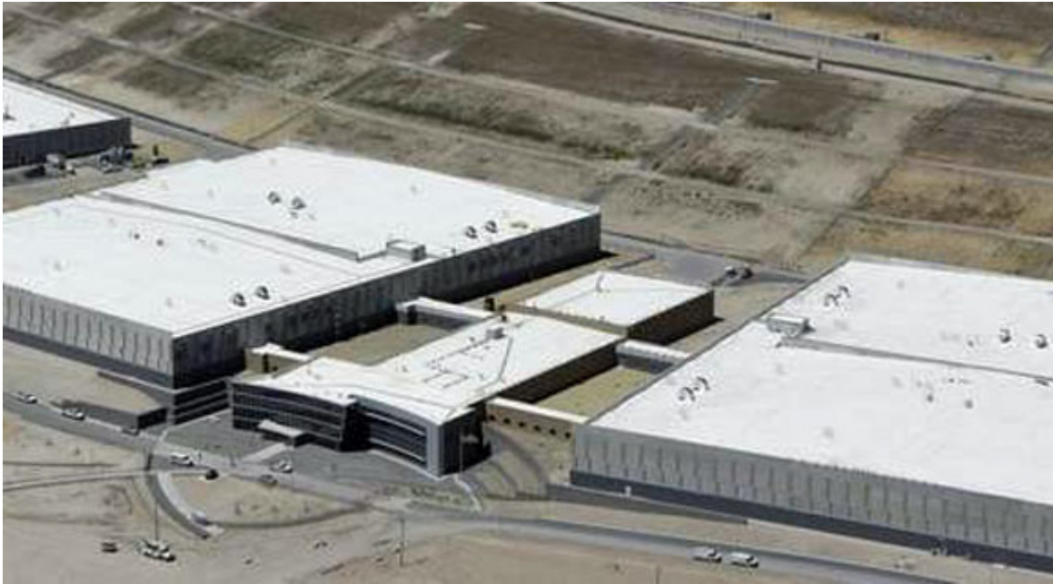
• Four completed data halls and the Administration building - June 2013
