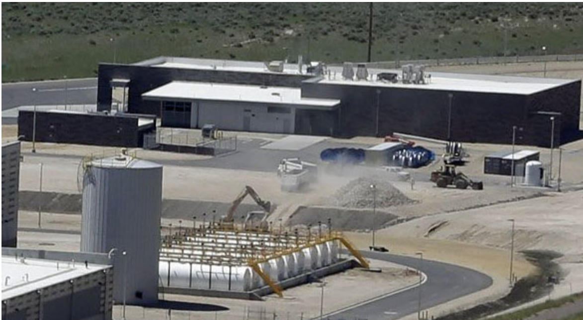
• Storage warehouse, canine kennel, and sprinkler system water tank - June 2013
