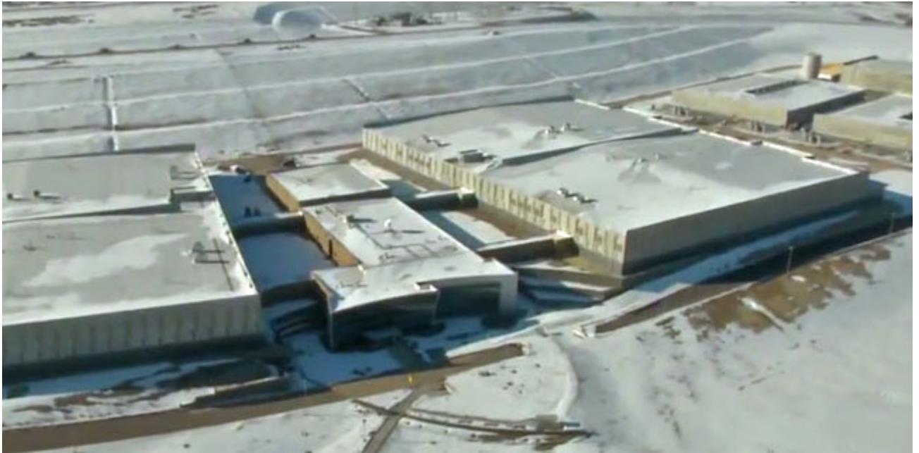
• Administration building and our four data halls
