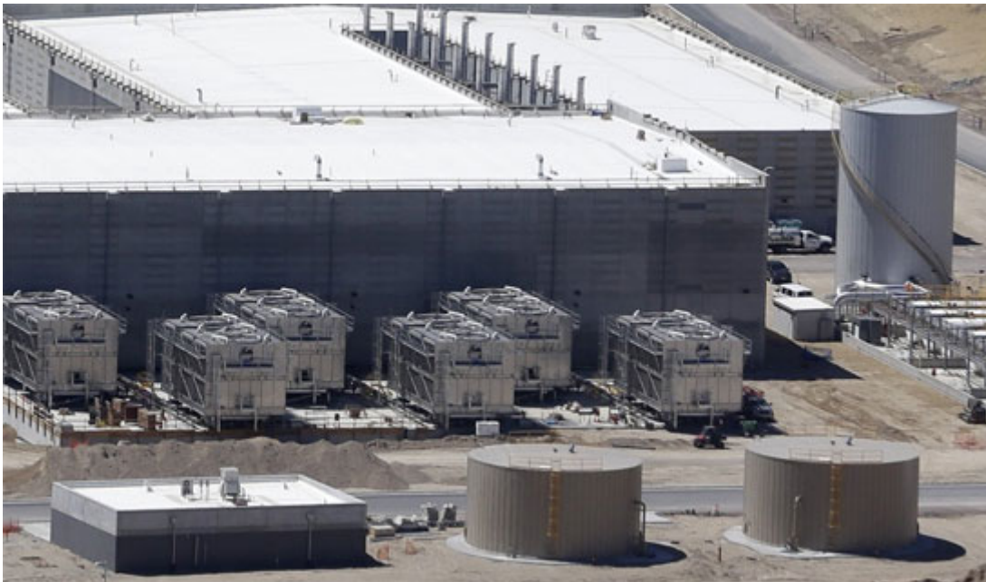
• Completed chiller/generator plants and fuel tanks - June 2013
