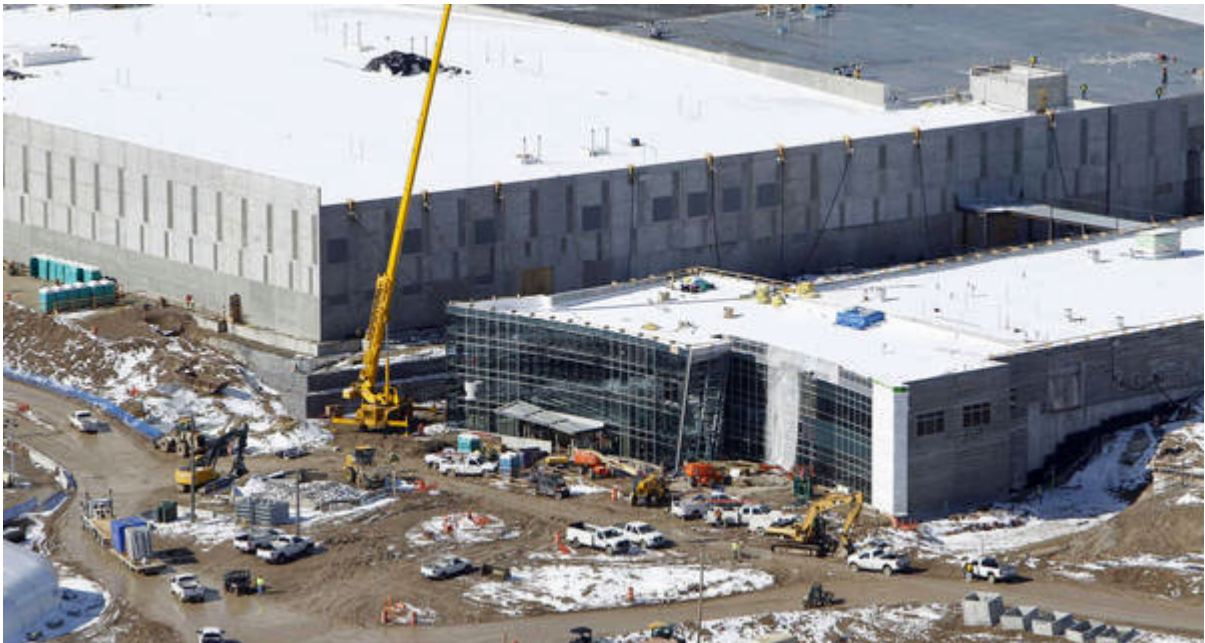
• Close-up view of a data hall and the Administration building - March 2012
