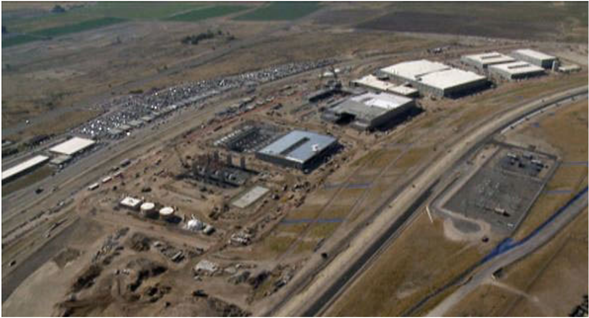
• Aerial view of the UDC construction site - July 2012
