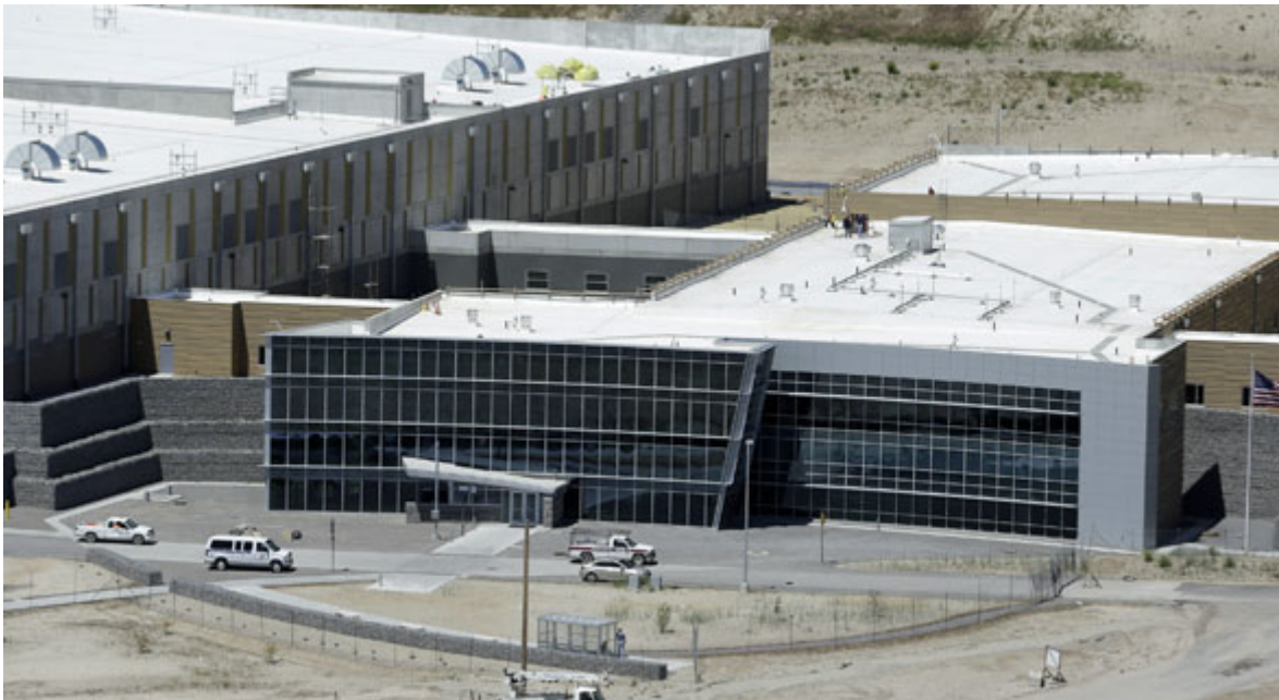
Close-up view of completed data hall and Administration building - June 2013
