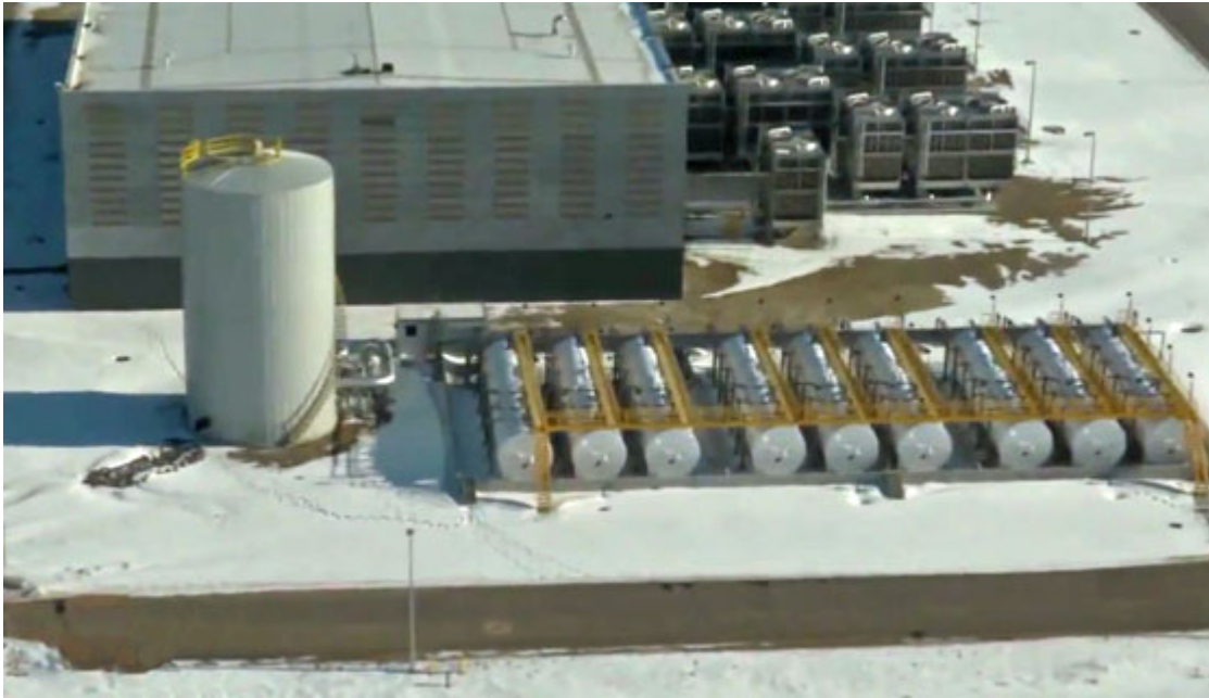
• Water tanks for our chiller plant
