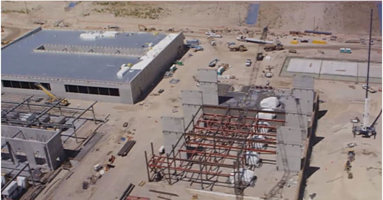
Chiller plant, generator plant, and tank storage under construction - July 2012
