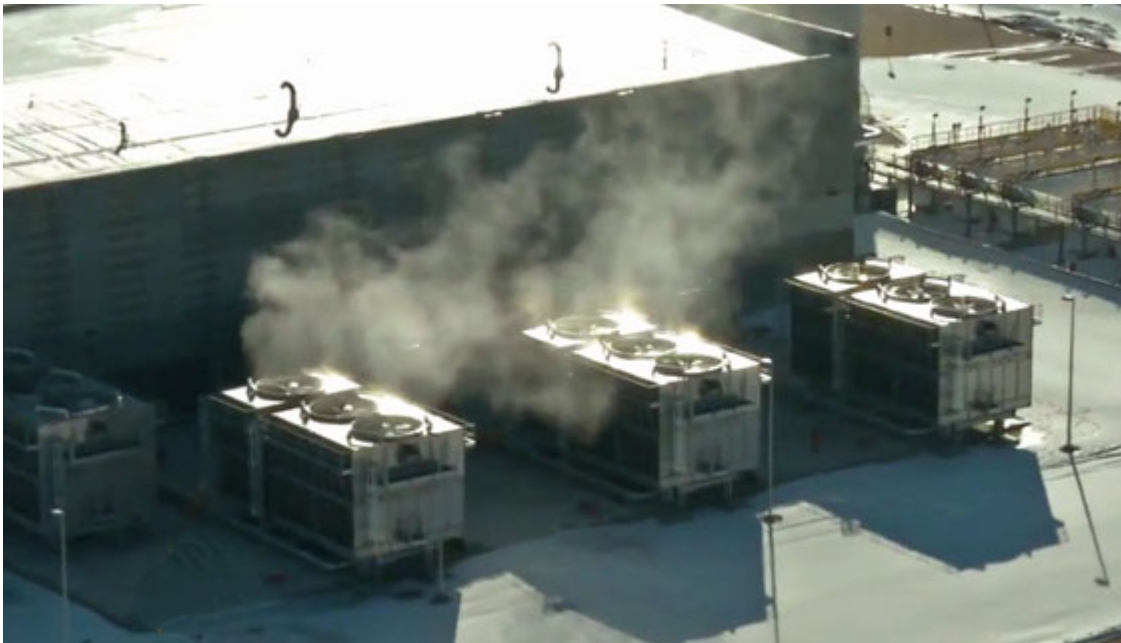
Our massive cooling systems at work
