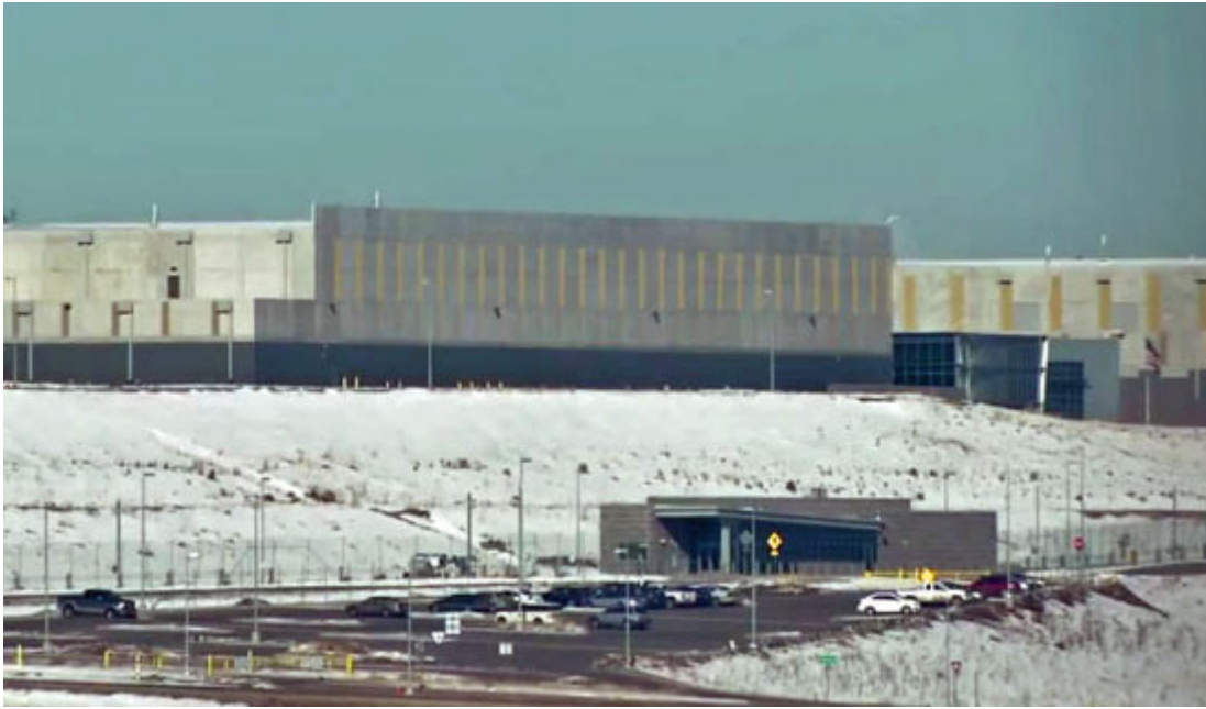
Visitor Control Center
