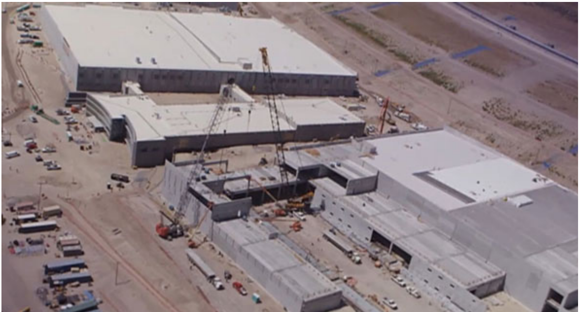
• Last two data halls still under construction - July 2012
