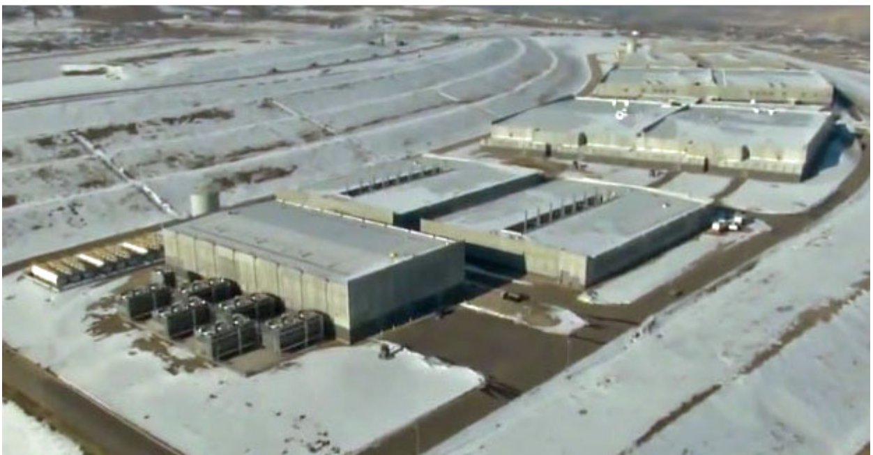
• Chiller plant and generator plant
